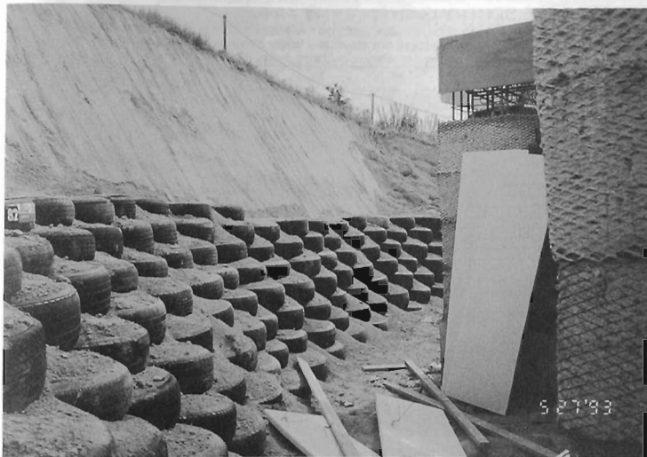
TIRE RETAINING WALL BEHIND EARTHSHIP IN JAPAN.
