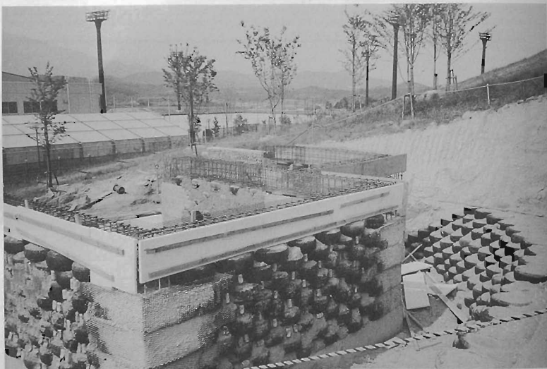
EARTHSHIP IN JAPAN SHOWING KNITTED IN CONCRETE POST AND BEAM FOR EARTHQUAKE DESIGN
