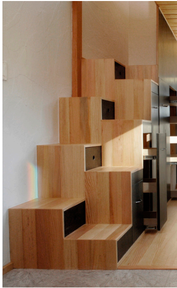
An example of stairs using alternating tread devices in a tiny house built by Chad Smith of StructuralSpaces.com. Photo by Jenn Walton/Digiwerx Studios
