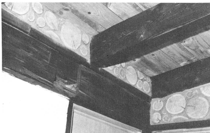
Fig. 95. Log-ends fill the space between rafters from the top of the beam to the roof planking and go well with the rough-hewn style of the house.
