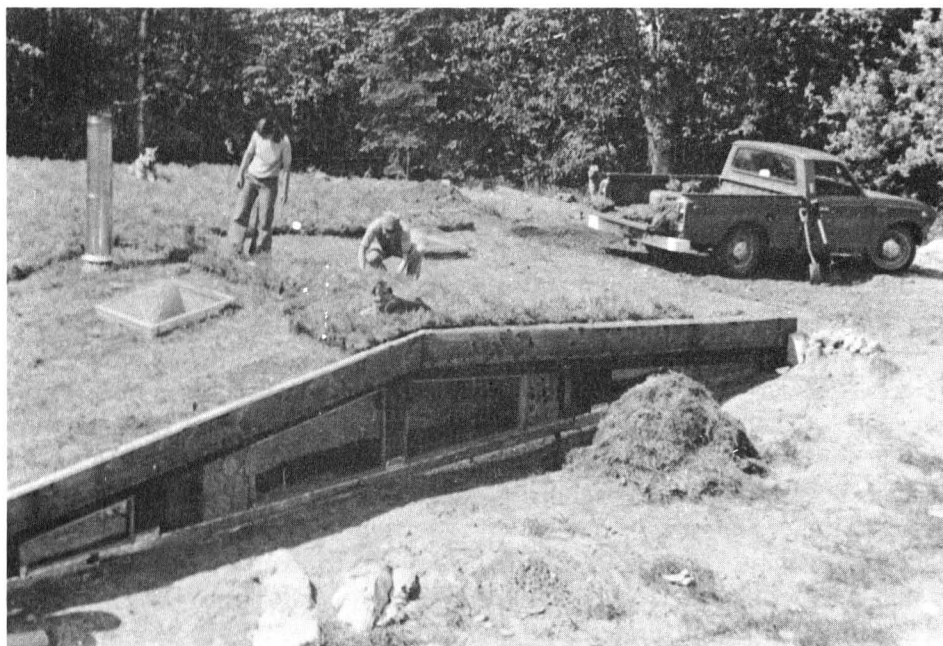
Fig. 73. Laying sod is easy: with the side of your foot, simply kick each new piece against those already laid.
