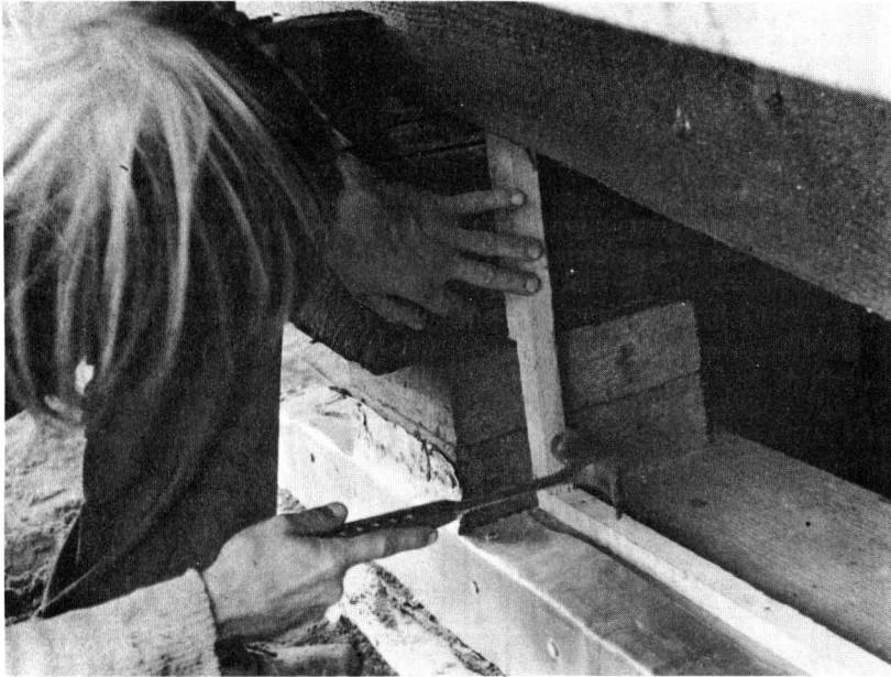
Fig. 76. Preparing to install the trapezoidal window in the north wall.
