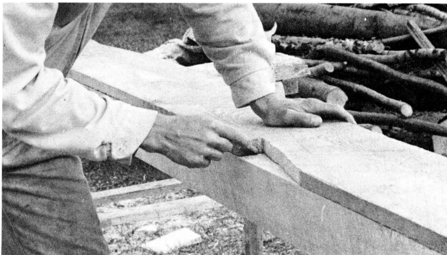
Fig. 48. Using a template will ensure correct marking for the birdsmouths on each rafter.
