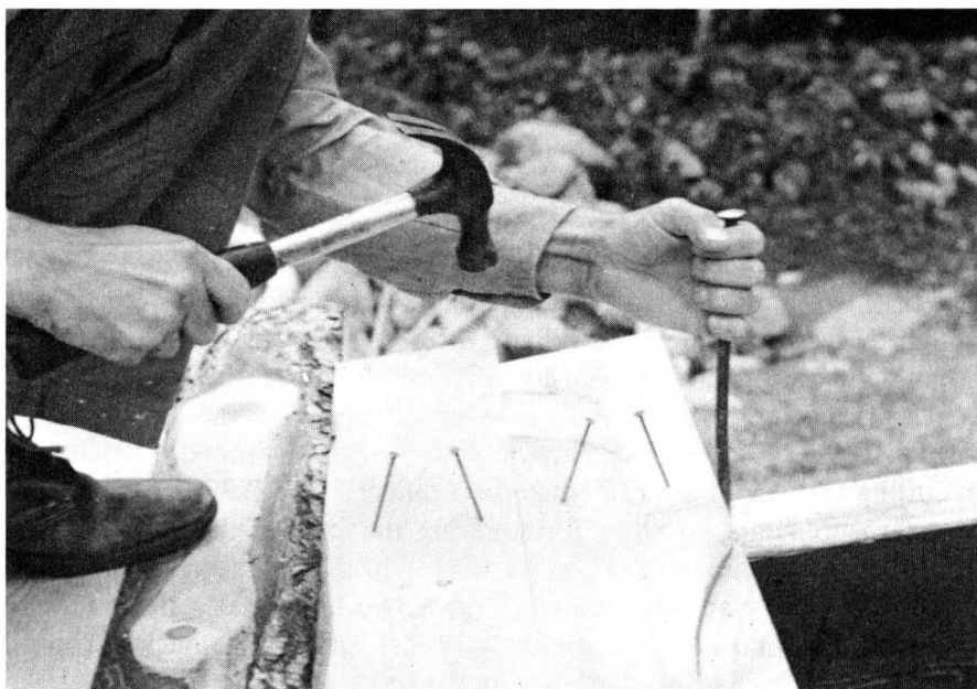
Figs. 52 and 53. If you are using green wood, nail the planks as shown here, using a spike to keep them tight against each other and nailing the lower nails first.
