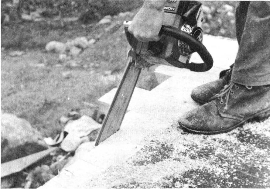
Fig. 56. Leave the plank ends sticking out; the overhang can be trimmed later by snapping a chalkline and cutting the whole edge at once.
