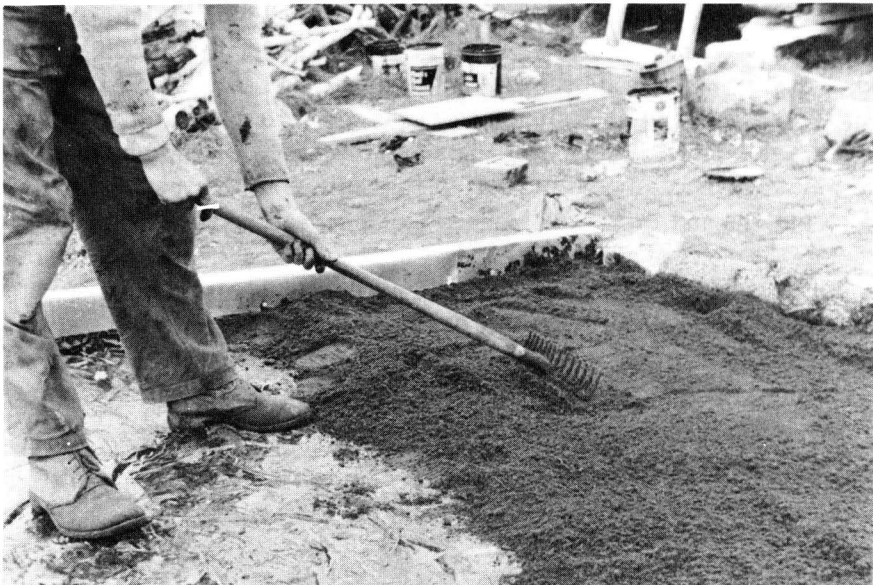
Fig. 72. A 4-inch layer of topsoil covers the roof.
