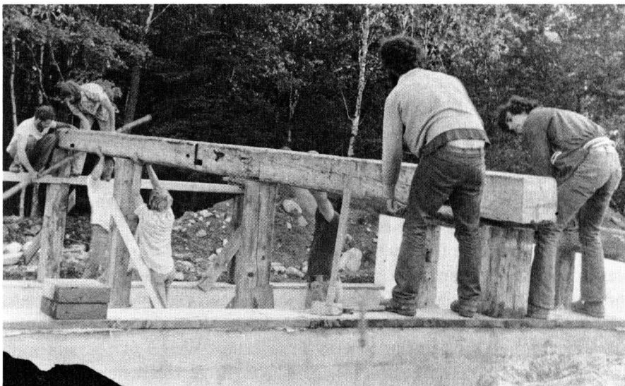
Fig. 44. The beam was then cantilevered over the north wall and positioned on the posts.
