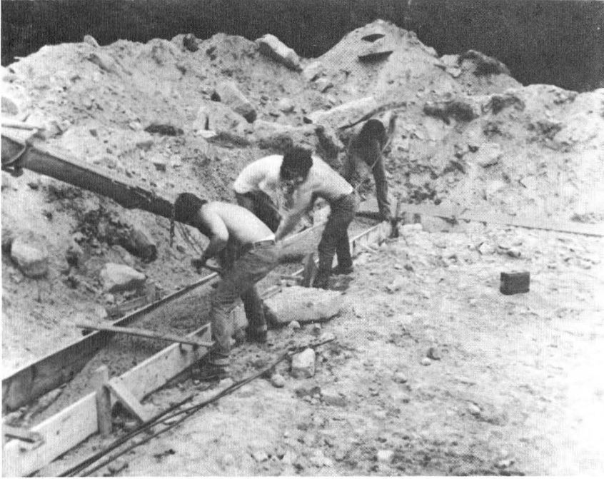
Fig. 18. A crew of four or five, each with a good, strong rake, should be sufficient to draw the concrete around the footing ring.
