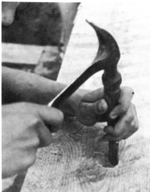
Figs. 37, 38, 39 and 40. After the anchor bolts have set in the concrete, locate the holes in the plate by laying the plate on the anchor bolts and whacking once sharply with a sledgehammer. The indentations in the plate mark the locations of the holes to be drilled. Turn the plate upside down and drill holes the same diameter as the bolts. Chisel out a depression to accommodate a washer and nut.
