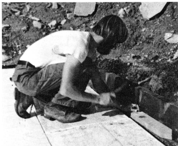
Fig. 58. Fascia boards were fastened by first nailing a 2-by-6 plank along the edge of the roof, then nailing scraps of economy-grade 2-by-4s on top of the plank.
