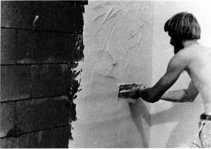
Fig. 35. Work the mix onto the wall with a plasterer's trowel.
