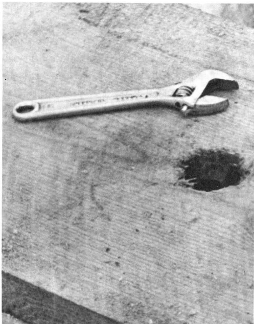
Figs. 37, 38, 39 and 40. After the anchor bolts have set in the concrete, locate the holes in the plate by laying the plate on the anchor bolts and whacking once sharply with a sledgehammer. The indentations in the plate mark the locations of the holes to be drilled. Turn the plate upside down and drill holes the same diameter as the bolts. Chisel out a depression to accommodate a washer and nut.
