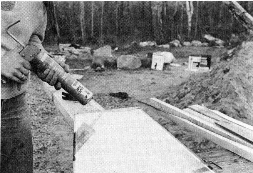
Fig. 75. Double-caulk the windows by running a bead of silicone along the glass itself and another bead along the molding surface to be placed against the sill or lintel.
