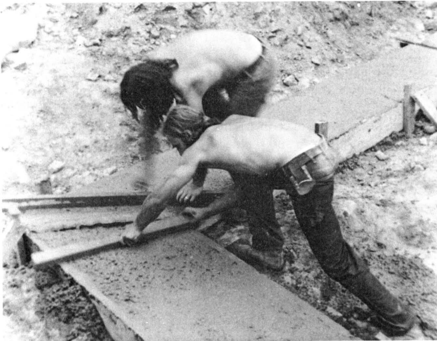
Fig. 20. The concrete can be screeded (made level with the top of the shuttering) with 2-by-4s.
