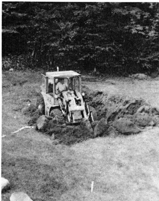
Figs. 10. and 11. Excavating into a hillside is easier with a front-end loader and its 6-foot bucket. The site should be excavated to a flat surface about 2 feet beyond the outside of the planned footing.
