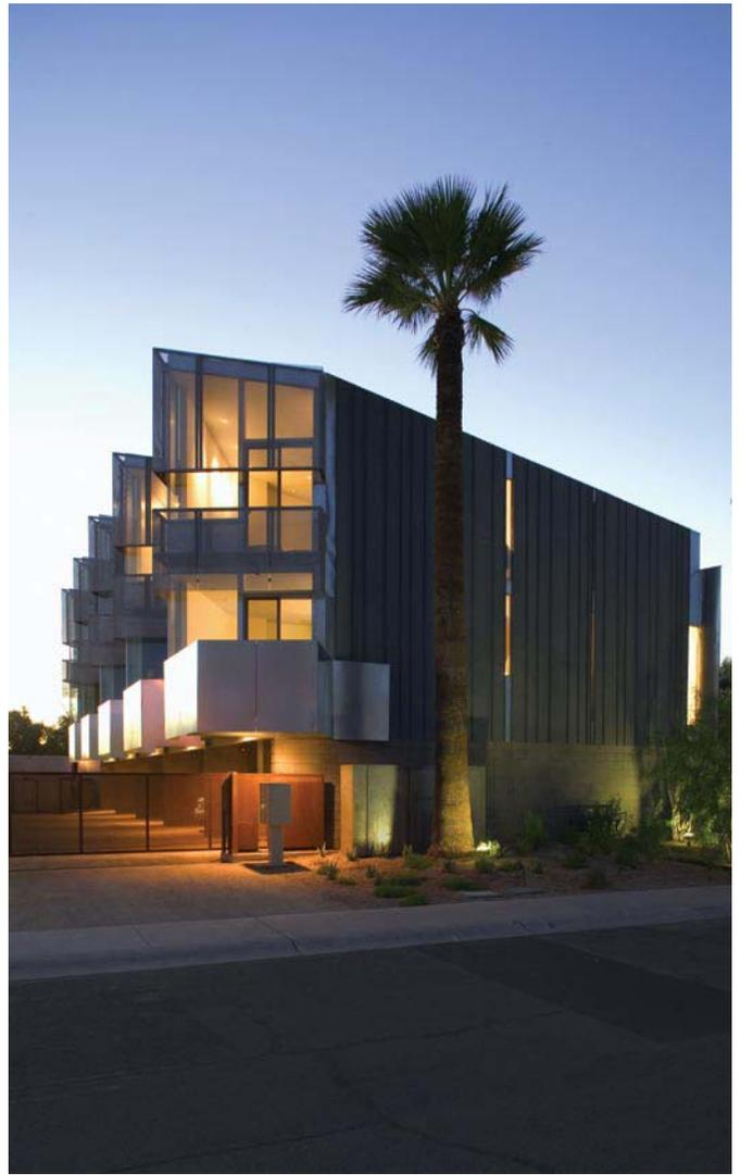
windows are substantially covered with perforated metal scrims, which are about 70 percent solid and 30 percent void. The scrims cover the upper half of the second-story windows and most of the windows on the third floor.
