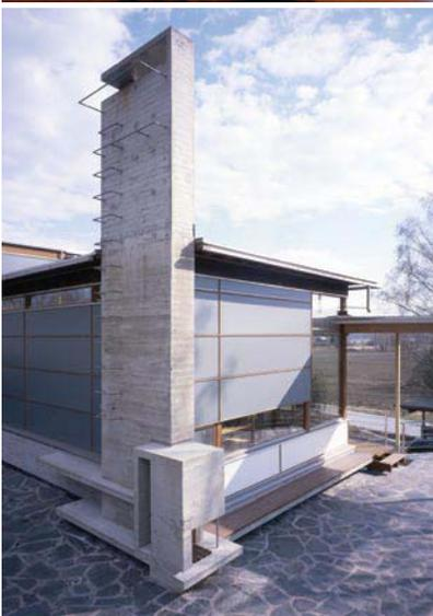
↔ An ambitious circulation scheme allows heat from the fireplace to flow throughout the interior. The windows' interior reflective coating keeps heat from escaping during the winter.
