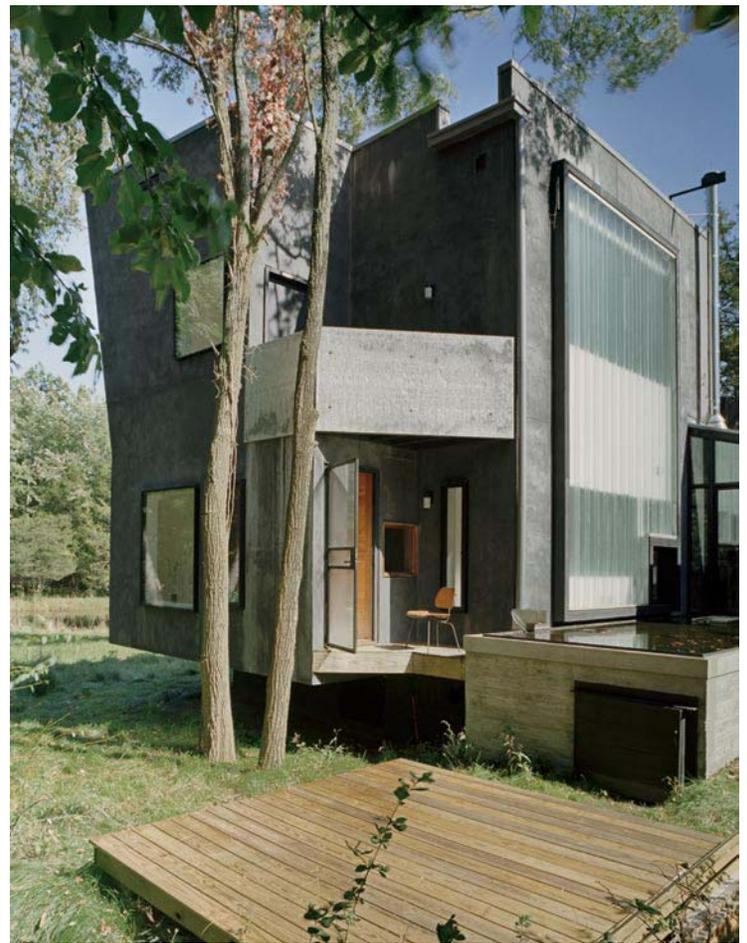
← The two-story addition is made up of a warped cube covered with charcoal-gray stucco and punched through with steel-frame windows.
