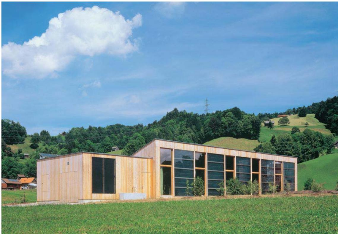
← The roof of the house slopes up, allowing the southern facade to be as tall as possible. Glass panels alternate with bands of Power Glass, a material Schwarz invented, to catch and store the winter sun.
