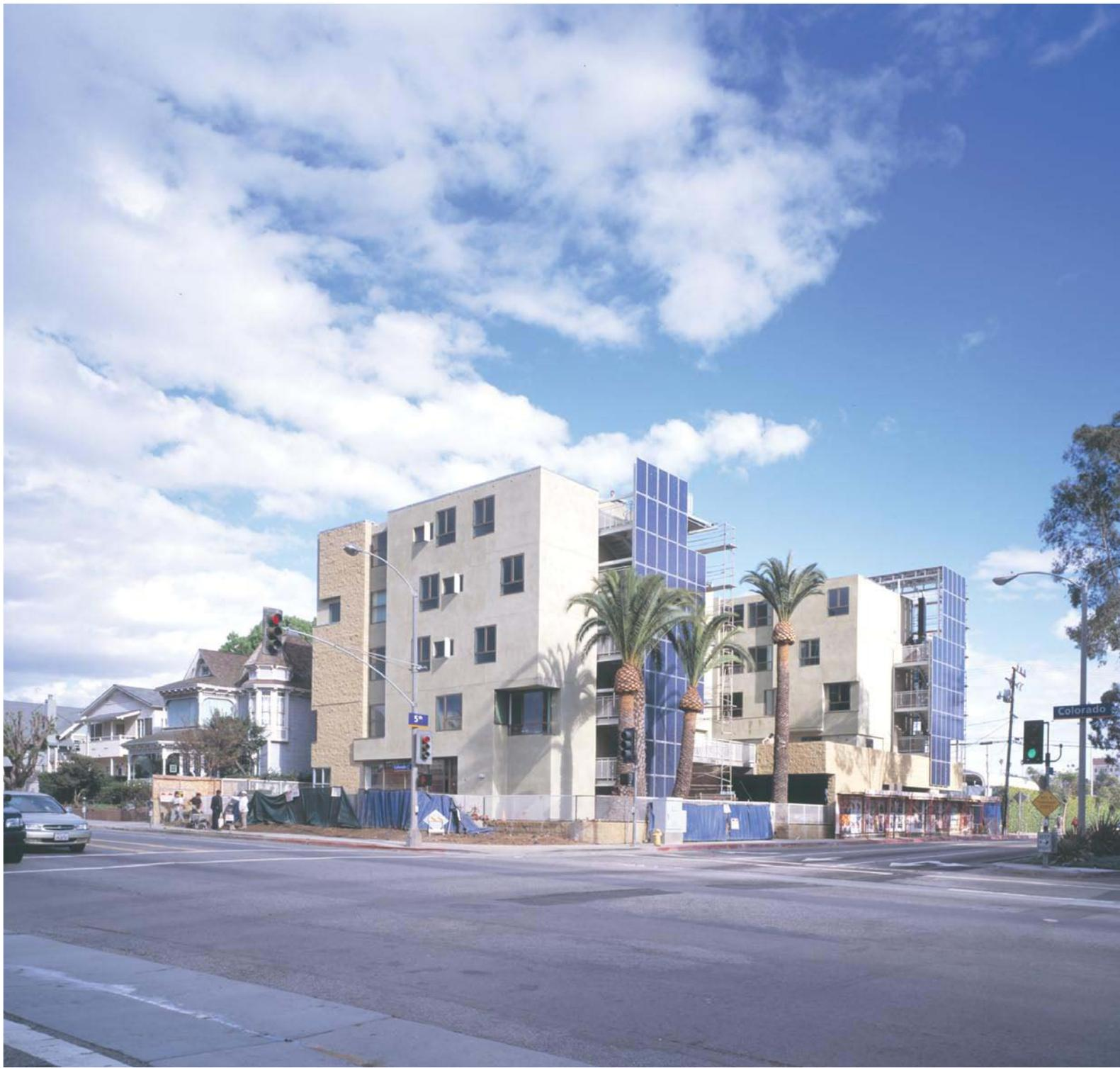
→|→ The 199 photovoltaic panels covering the facade (and portions of the roof) represent a rare effort to turn solar power into an aesthetic virtue. The 5-by-5-inch panels generate more than 90 percent of the building's electricity needs.
