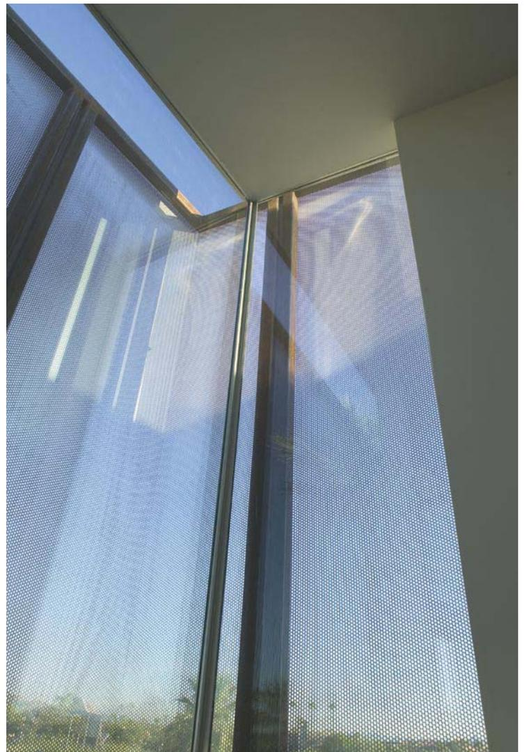
↑↗ The windows on the northern side of the building are partially enclosed inside perforated metal screens that help reduce glare and solar gain. Seen from inside, the screens maintain a surprising degree of transparency.
