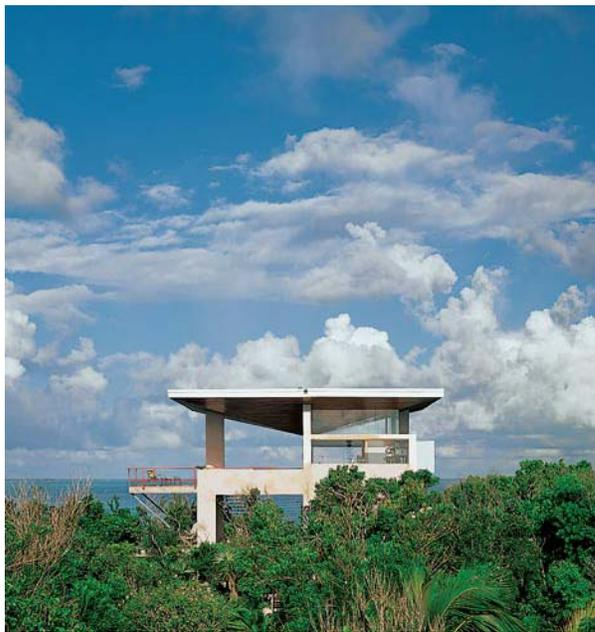
↑ Pitched downward beneath a flat topline, the angled roof is designed to collect rainwater and then funnel it down to an 8,000-gallon cistern.
