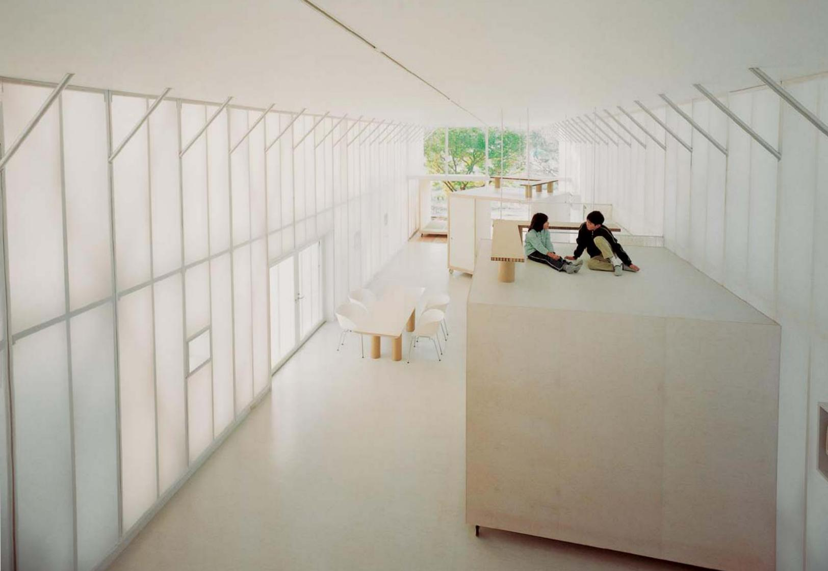
↑ Set into basic wood stud frames, the wall panels are made of corrugated plastic on the exterior and lined with nylon fabric on the inside. Clear plastic bags stuffed with polyethylene foam inserted in between serve as insulation.
