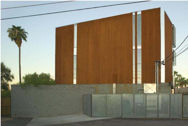
↑↑ The western facade is faced in Rheinzink panels sliced through vertically with narrow windows.
