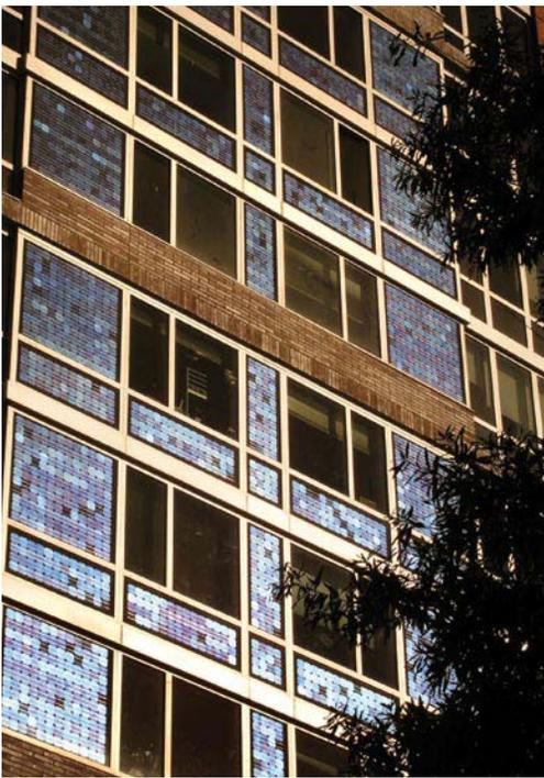
↑ With 3,400 square feet of photovoltaic panels, among other energy conserving elements, the Solaire uses 67 percent less electricity during peak hours than comparable buildings.
