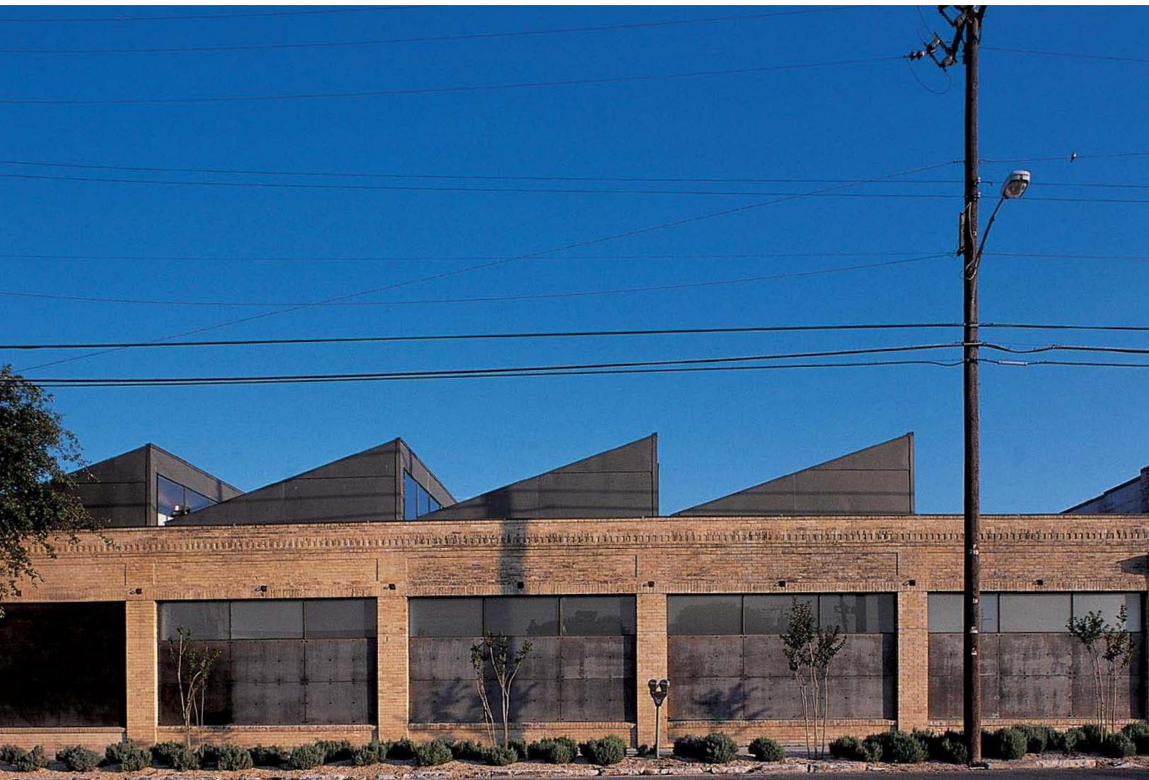
↑ Black-painted concrete fiberboard (a sturdy blend of recycled paper, cement, and concrete) set into the original brick structure preserves the building's industrial character from the outside, while ensuring privacy and security for the owner on the inside.
