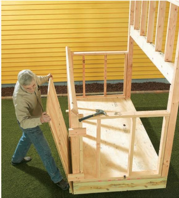
**6** Nail the exterior siding to the framing for the front wall. The top edge should be lower than the top of the 2 × 4 framing to leave room for the glazing overhang. Nail temporary stops at the corner to help position the siding.
