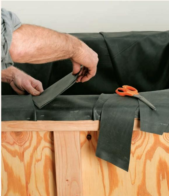
**11** Level out the rubber ledge between the corner folds with scrap pieces of rubber.
