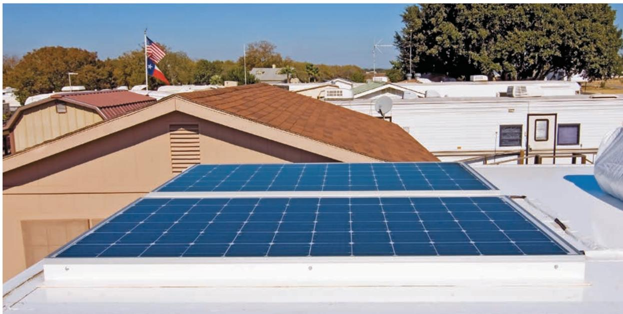
Rigid solar modules are durable and efficient, which makes them a good choice for RVs with a flat roof. Flexible modules that are very thin ( $\frac{1}{8}$ " ) and flex to follow a profile up to 30° make sense atop some RVs that have round roofs.
