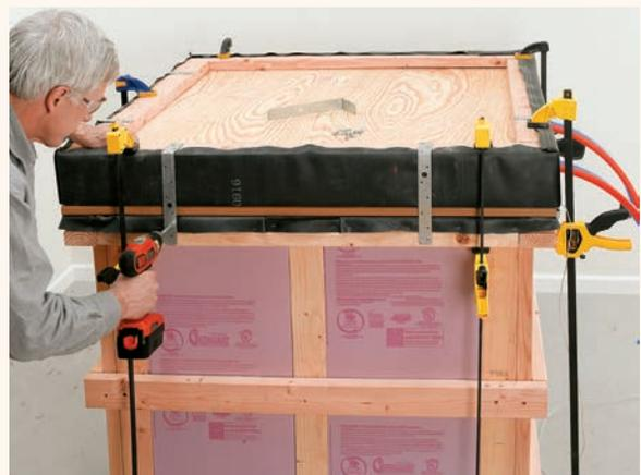
**17** Complete the plumbing connections inside the tank, fill gaps around the pipes on the ledge with silicone, then clamp the top down tightly to seal the edges. Fasten the top to the base with galvanized straps and deck screws.
