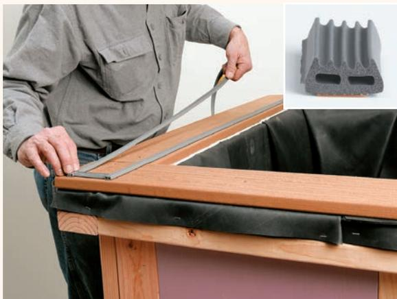
**16** Add two strips of weatherseal on the ledge about 2" apart. Use a soft foam type that compresses easily and fills voids, like this (inset).
