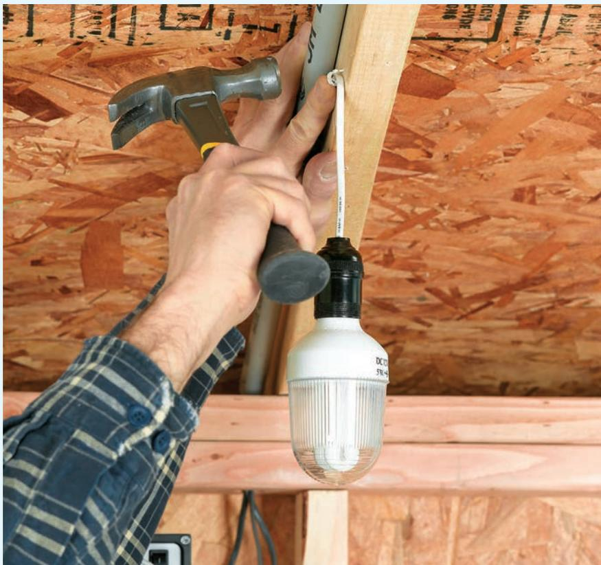
**10** This kit includes two DC lights. To install them (or other DC appliances), just plug the cord in to the proper port (or adapter) and turn the power on. Hang the 12-volt light fixtures from the rafters and then staple the cords to keep them secure and out of the way. Make sure to leave enough cord that the plug end is easy to insert and remove from the port. You'll plug and unplug the lights to turn them on and off.
