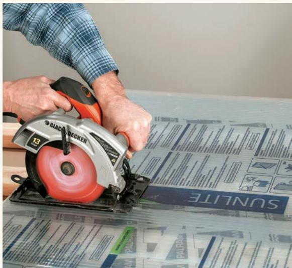
**10** Cut the polycarbonate glazing so that it matches the width of the box. Cut it long enough so it tucks under the overhang at the top and hangs over  $\frac{1}{2}$ " at the bottom. Make sure to install it with the UV-protected side up (the side with the label).
