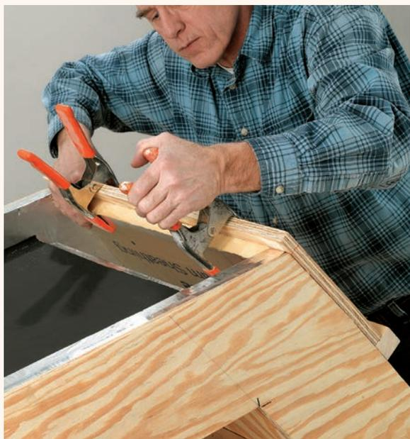
**9** Cut and install 1" polyiso insulation to fit the angled top, from the  $2 \times 2$  to the outside corner. Caulk any gaps along the sides. Spread a bead of glue on the insulation, then cover it with  $\frac{3}{4}$ " plywood screwed across the top, and extending from the  $2 \times 2$  to 1" beyond the outside corner. Clamp the plywood and insulation until the glue sets.
