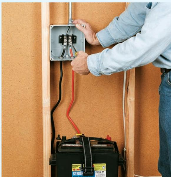
**14** Install the battery. Here, a deep-cycle 12-volt marine battery is used. First, cut and strip each of the two battery cables at one end and install into the battery control junction box through cord cap connectors. Terminate these wires on two separate, firmly mounted insulated terminal blocks.
