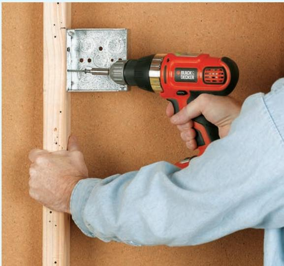
**3** Attach a junction box for enclosing the DC disconnect, which is a heavy-duty switch, to a wall stud near the battery and charge controller location. Use a metal single-gang box with mounting flanges.
