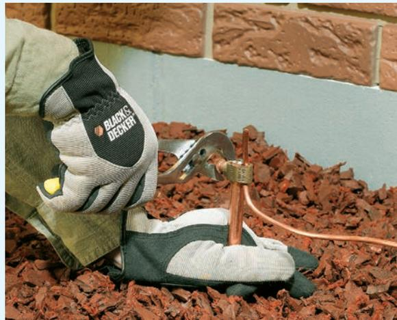
**10** Set up grounding protection, if required. Pound an 8-ft.-long, 1/2"-dia. ground rod into the ground outside the building, about 1' from the wall on the opposite side of the charge controller. Leave about 2" of the rod sticking out of the ground. Attach a ground rod clamp to the top of the rod. Drill a 5/16" hole through the garage wall (underneath a shake or siding piece) and run the #6-gauge THWN wire to the ground rod. This ground will facilitate lightning protection.
