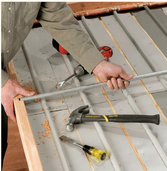
**12** Create cross-bar supports for the polycarbonate glazing by installing two lengths of  $\frac{1}{2}$ " EMT conduit across the box. Drill  $\frac{3}{4}$ " holes halfway through the 2 x 4 sides, centering the drill bit  $\frac{3}{8}$ " down and drilling from the inside. Square the holes with a chisel, then place the conduit in the holes.
