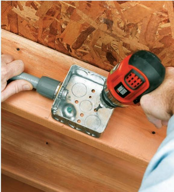
**1** Mount a junction box inside the building where the conduit enters from the module. Secure the conduit to the box with appropriate connectors. Run two 14-gauge wires through the conduit, leaving excess at the module and junction box. *OPTION: Using PVC conduit and electrical boxes instead of metal can reduce labor and materials costs and eliminate the need for grounding the metal conduit.*
