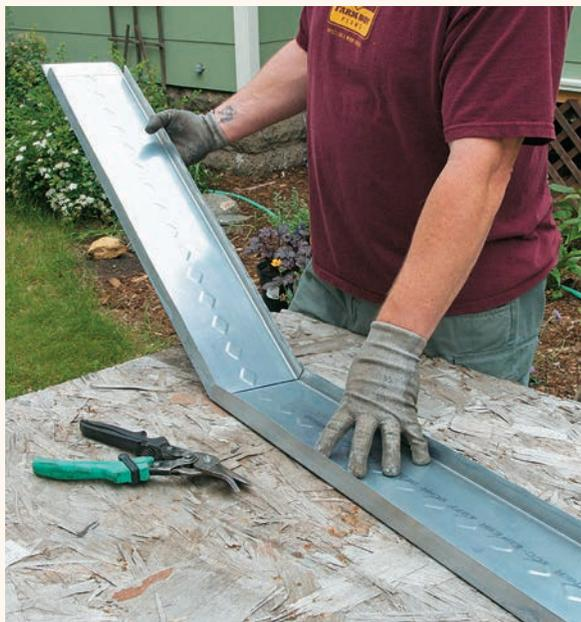
**1** Cut and bend the box frame pieces from 2 × 6 steel studs. Each steel stud piece will wrap two sides of the panel with a 90° corner bend. Mark the bend location on both steel studs. Cut a relief into the 6" side of the stud with aviation snips at this mark. Bend the stud to an L-shape and use a square to ensure that the corner forms a true 90° angle.
