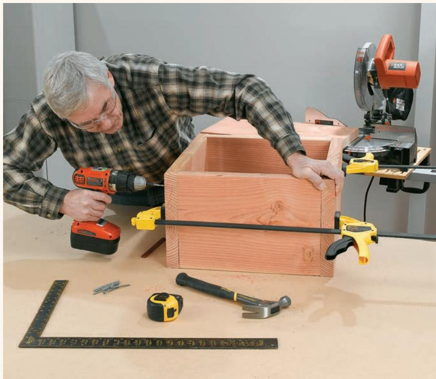
**1** Cut the four 2 × 12 base pieces to length according to the cutting list. Arrange the base parts on a flat work surface and clamp them together in the correct orientation. Check with a carpenter's square and adjust the parts as needed. Then drill pilot holes and fasten the pieces together with 2½" deck screws.
