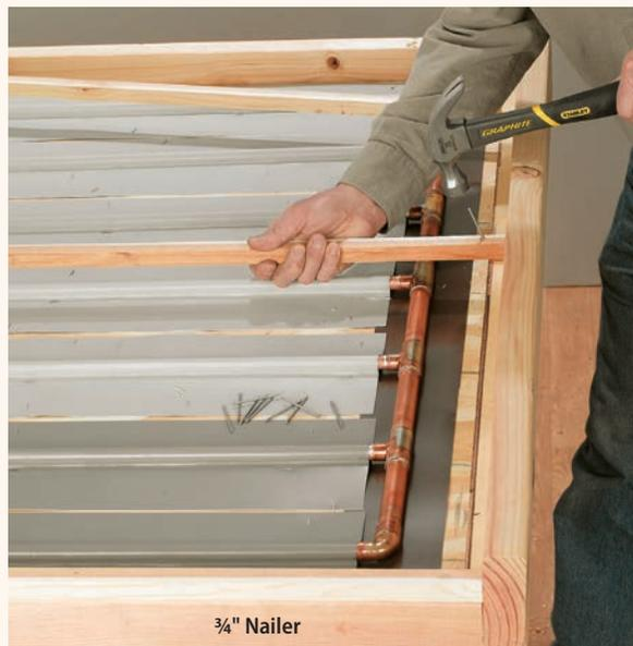
**13** Lay the glazing on top of the box and mark the spots for  $\frac{3}{4}$ " nailers at the sides and the center overlap. Fasten the strips with 6d galvanized casing nails.
