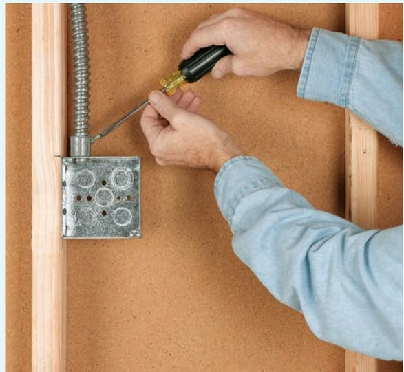
**4** Run flexible metal conduit from the entry point at the power source to the junction box for the DC disconnect box. Use hangers rated for flexible conduit.
