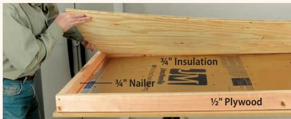
**4** Cut panels of ¾"-thick closed-cell, foil-faced polyiso insulation and fit them inside the frame between the ¾" nailers, flush with the tops of the nailers. Cut a panel of ½" plywood to fit inside the frame over the insulation and the nailers and attach the plywood to the nailers, driving a 1¼" screw every 10" to 12" around the perimeter. Caulk the gap between the ½" plywood and the frame with clear, 100% silicone caulk.
