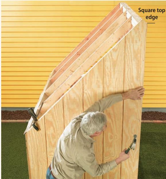
**12** Install exterior siding on the walls and doors and above and below the doors. Square off the top end of the side piece as shown so it lines up with the 2 × 4 top plate and creates a small roof profile.
