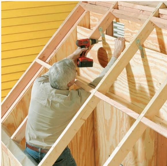
**16** Cut the shroud that the fans are attached to from  $\frac{3}{8}$ " or  $\frac{1}{2}$ " plywood. Attach 2 × 4 nailers to the sides (hidden behind the shroud in this photo), and screw a 2 × 4 across the bottom. Make cutouts for the fans you buy, then hang the shroud from the rafters with hurricane ties and screw the 2 × 4 to the side walls. (Fans can be any inexpensive type, 8" to 14" round or square, as long as you can find a way to fasten them.)
