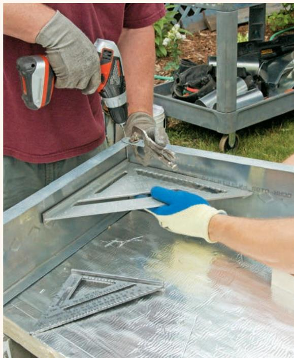
**2** Drill 1/8"-dia. holes in the overlapping top and bottom flanges. Clamp the corners together before drilling, using a square to make sure the corner forms a 90° angle.
