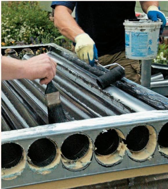
**11** Paint the last section of ductwork and touch up around the interior of the box so all exposed surfaces are black.
