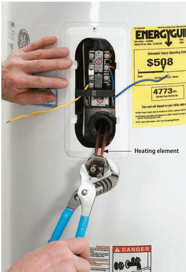
Turn off and disconnect any wiring to the heater you'll be converting to a storage tank. Remove the covers over the heating elements, cut away the wiring, then turn out both heating elements with a socket wrench or a channel lock wrench.
