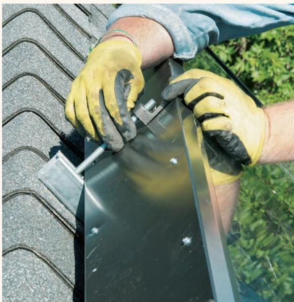
**19** Connect the panels to the Unistrut with a  $\frac{3}{8}$ " threaded rod attached at the top and bottom of the panel on the outside. Cut threaded rod to size, then attach to the Unistrut with Unistrut nuts. Attach the top clip to the top of the rod and the front face of the panel. Tighten the assembly to compress the panel down to the Unistrut for a tight hold.
