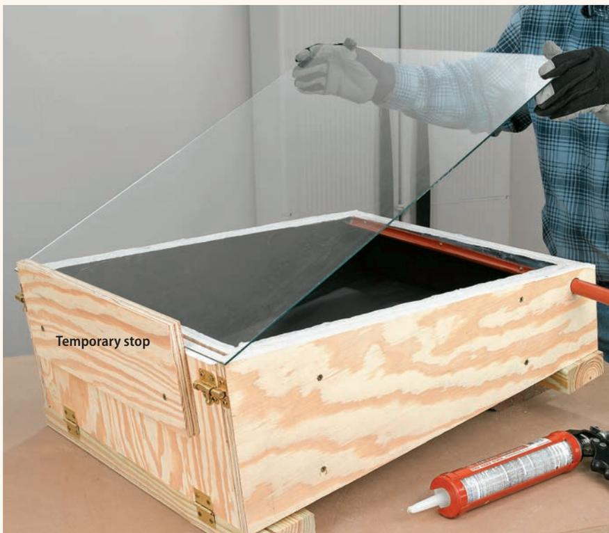
**12** Shim the box level and tack a temporary stop to the top edge to make it easy to place the glass without smearing the caulk. Spread a generous bead of caulk on all the edges, then lay the glass in place. Tape it down around the edges with painter's tape, then let it set up overnight.
