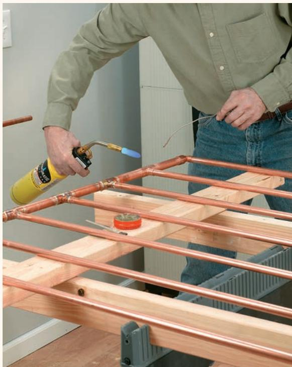
**6** Solder all the pieces together. Protect the floor from drips of solder and flux with a dropcloth. Wait at least 5 minutes to touch the copper after soldering it—it will be very hot.
