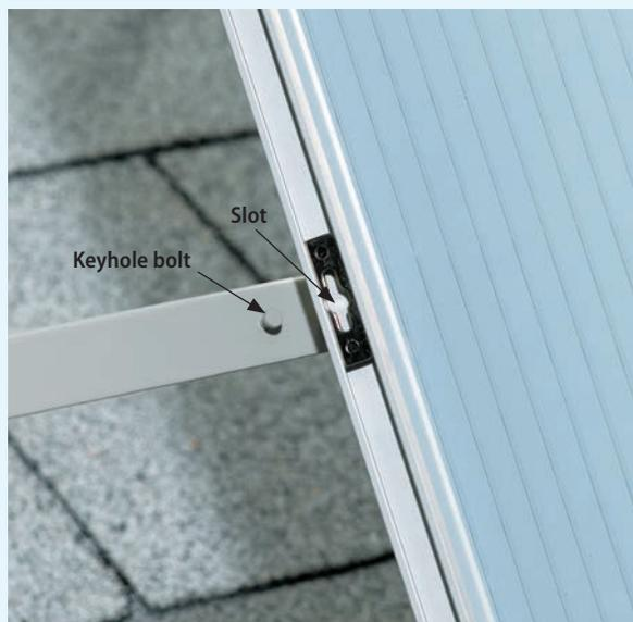
**4** Lock the PV panel down into position by sliding the small bolt heads on the brackets into the keyhole slots on the back of the panel. (Other kits may use different fasteners.) Cover the panels with a drop cloth after they're in position—they'll start generating electricity as soon as the sun hits them.
