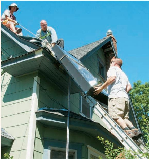
**17** Hoist the panels into position. Carefully follow safety regulations and use scaffolding, ladders, ropes, and lots of helpers to hoist the panels onto the roof. Wear fall-arresting gear and take care not to allow the plenum ductwork to be damaged.
