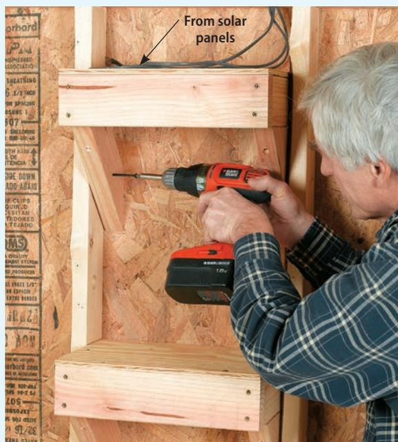
**7** Install two sturdy shelves inside the building to hold the regulator and the battery. The shelf should be reachable by an adult so the equipment can be turned on and off and plugged into the adapter easily. The battery shelf should be at least 18" off the ground.
