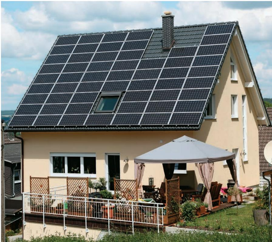
This house is still connected to the electrical grid, but with the entire south side of the roof covered with solar panels, the homeowner generates enough electricity on sunny days to earn money back from the utility company.
