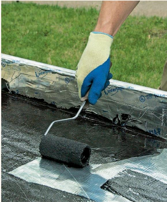
**9** Paint the entire box interior using black high-temperature paint and allow it to dry completely. A trim roller works well for this task.
