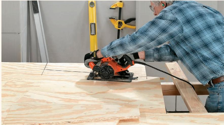
**2** Cut the insulation the same size as the plywood base, then screw both to the 2 × 4 supports with 2½" screws.
