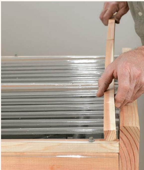
**16** Cover the ends of the glazing with  $\frac{3}{4}$ " wood strips. Predrill and fasten the strips with  $2\frac{1}{2}$ " deck screws. Caulk the strip at the top against the  $2 \times 6$  cap using paintable acrylic caulk.
