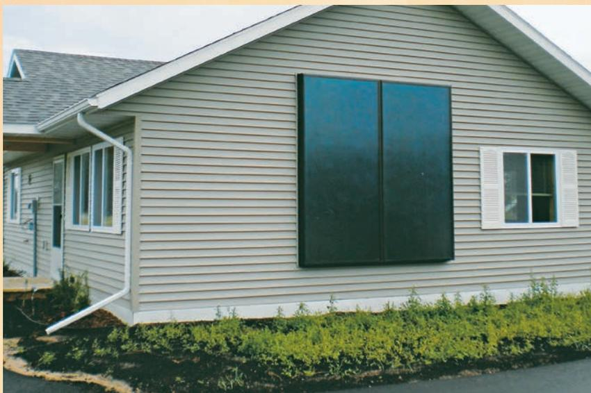
A solar air heater was built into the framing of the wall, with the siding trimmed around it (see Resources, page 186).
