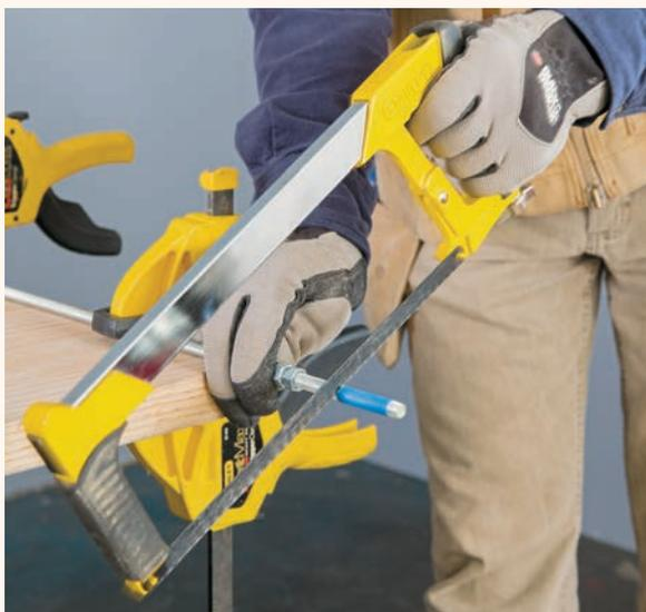
**11** Mark a length of  $\frac{5}{16}$ " threaded rod at 22". Thread two nuts onto the rod so they are about 18" from one end and both inside of the 22" mark. Cut the rod at the mark, using a hacksaw. Place a washer over the rod end, and insert it through the hole in the dish's center block, so the rod projects up out of the bottom of the reflective dish. Secure the rod on the backside of the plywood base with another washer and nut.
