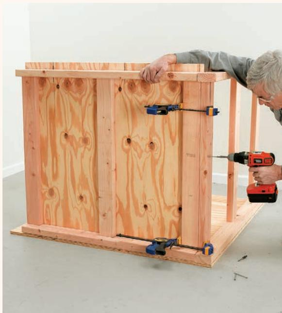
**3** Place the  $\frac{3}{4}$ " plywood base at the tank location, then connect the short sides to the long sides, fastening the overlapping corner 2 × 4s together with the long deck screws.
