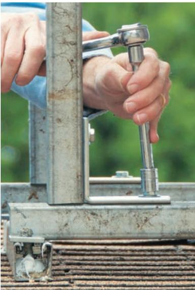
The stand components are held together with bolts and spring-loaded fasteners. The 45° and 90° connectors are manufactured specifically for use with this Unistrut system.
