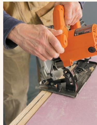
**2** Create the top channel by clamping an  $8' \times 2$ " to a work surface and drawing a centerline down the length of the board. Set a circular saw to cut a  $22\frac{1}{2}^\circ$  bevel at a depth of  $\frac{3}{4}$ ". Cut along the line, moving the clamps if necessary, to cut at least  $78$ " of channel. Test-fit a piece of corrugated plastic sheeting in the channel; it should slide in easily for a snug fit. If necessary, widen the channel as needed by making a second pass with the saw.
