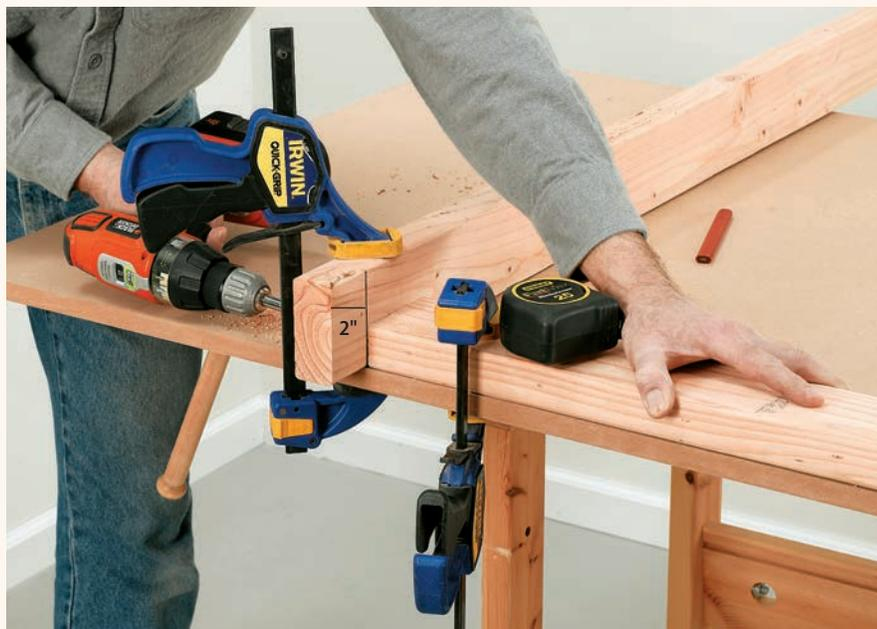
**2** Assemble the remaining sides, but instead of aligning the horizontal studs with the edge, fasten them 2" in from the edges. Place the third stud in the center.
