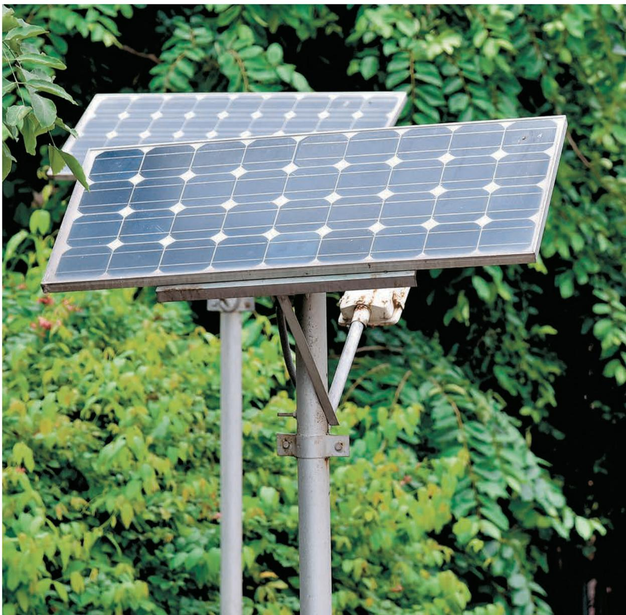
Mounting poles offer several advantages, but you must be sure that the poles are securely anchored in concrete and that the pole base is buried sufficiently deep.
