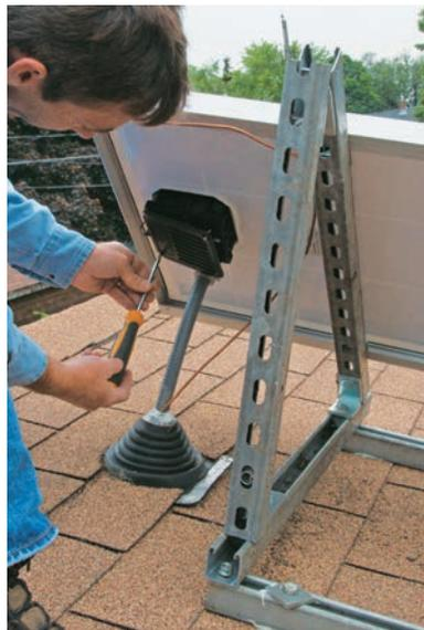
Connections for the feed wires that carry current from the collector are made inside an electrical box mounted on the back of the collector module.
