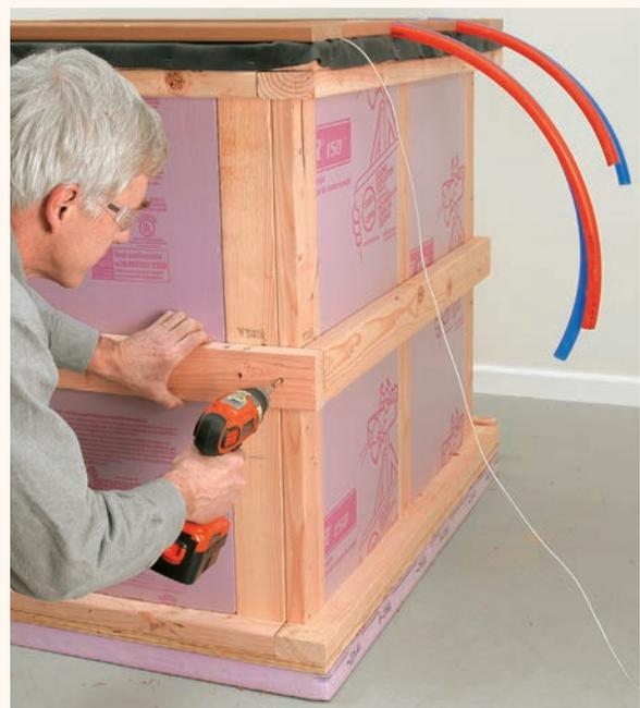
**14** Place  $1\frac{1}{2}$ " pieces of insulation on the sides, then install horizontal  $2 \times 4$ s around the center. If desired, you can add pieces of insulation above and below the  $2 \times 4$ s, then cover the sides with  $\frac{1}{4}$ " plywood for a finished appearance.
