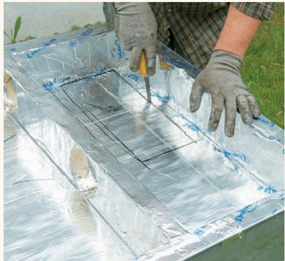
**8** Install a compartment separator in the first and last panels with a piece of foil insulation set on edge. Cut ductwork access holes in the separator. Then, cut out holes for the ductwork that will pass through the separator. Also cut a plenum opening in the separated compartment in the first and last unit.
