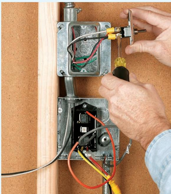
**11** Wire the DC disconnect. Attach the two #14-gauge wires to the two terminals labeled "line" on the top of the DC disconnect switch.
