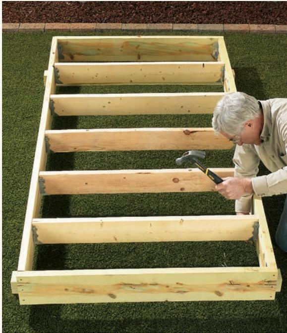
**1** Level a base of treated wood or concrete blocks at the kiln location, then build the frame for the floor on top of them. The kiln should be built in a south-facing location that gets at least five to six hours of direct sunlight.
