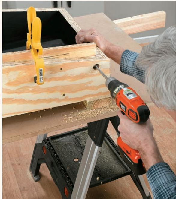
**8** Drill a hole for the PEX drain. The top of the PEX is  $\frac{1}{2}$ " down from the top edge. Clamp a piece of scrap wood to the inside so the drill bit doesn't splinter the wood when it goes through.
