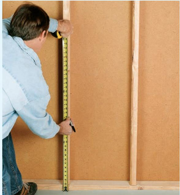
**2** Plan the system layout. Determine the placement of the battery and then decide where you will position the charge controller and DC disconnect. The battery should be placed at least 18" off the ground in a well-ventilated area where it won't be agitated by everyday activity. Mark locations directly on the wall.
