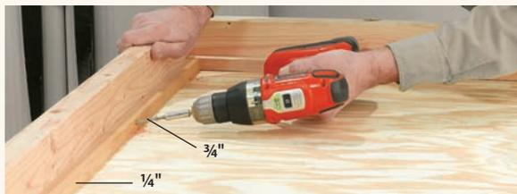
**2** Cut the ¼" plywood to size, then set it inside the frame as a spacer for the ¾" × ¾" nailers. If you can't locate ¾" × ¾" trim stock for the nailers at your building center, rip-cut ¾"-thick strips from a piece of 1× stock (a tablesaw is best for this, but you can use a circular saw and straightedge cutting guide, too). Screw the nailers to the inner perimeter of the frame with 1½" deck screws. Check to make sure the plywood is flush in back as you fasten the nailers.
