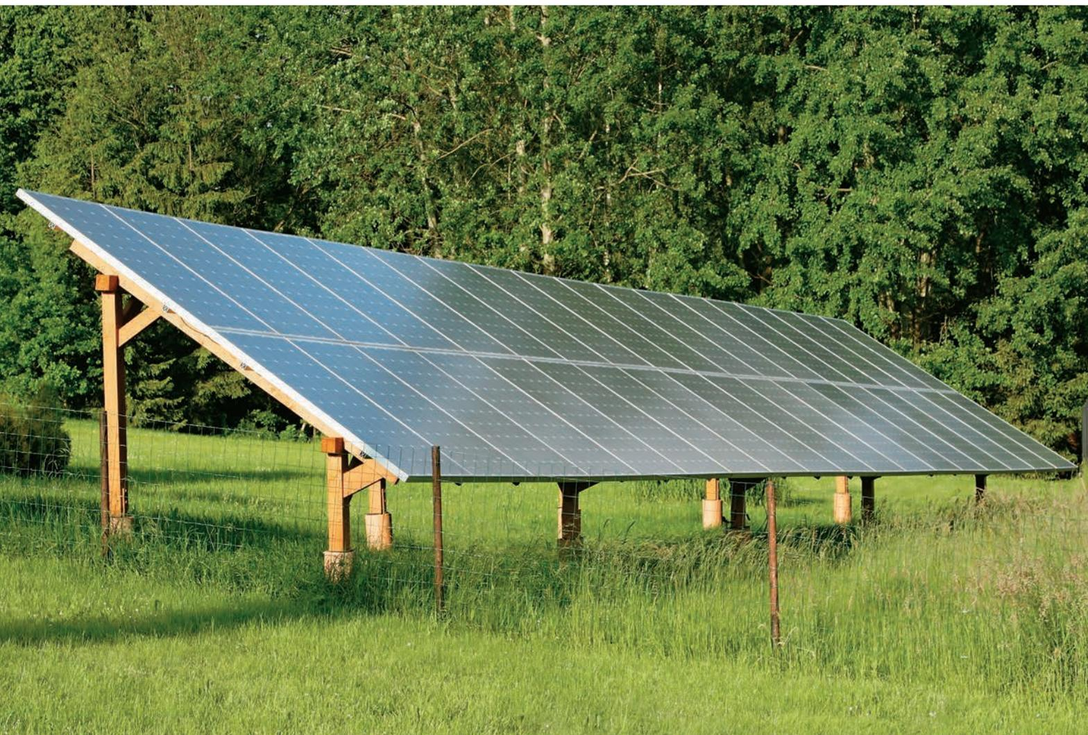
To protect against damage due to frost heave and ground movement, solar arrays must be set on poles that go down below the frost line. Some handy DIYers opt to use lumber for ground-mounting. Wood structures should be built with pressure-treated lumber and must be approved by the local building authority.
