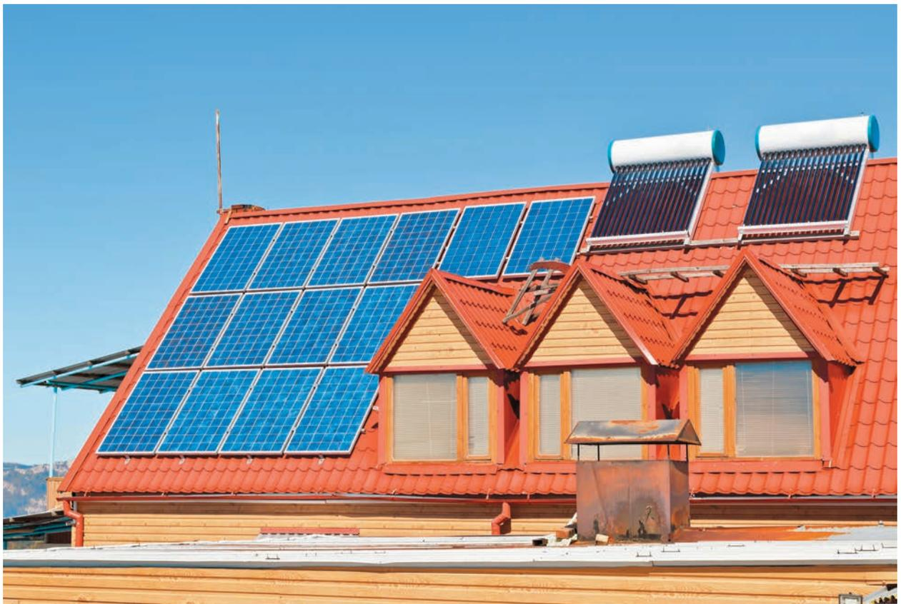
Combining solar thermal and PV systems once seemed like the ultimate way to go solar, but declining costs for solar electricity have made thermal systems hard to justify in many cases. It's often more cost-efficient to install a larger PV system and have it supply an electric resistance or heat pump water heater than to install a new thermal system for domestic hot water.
