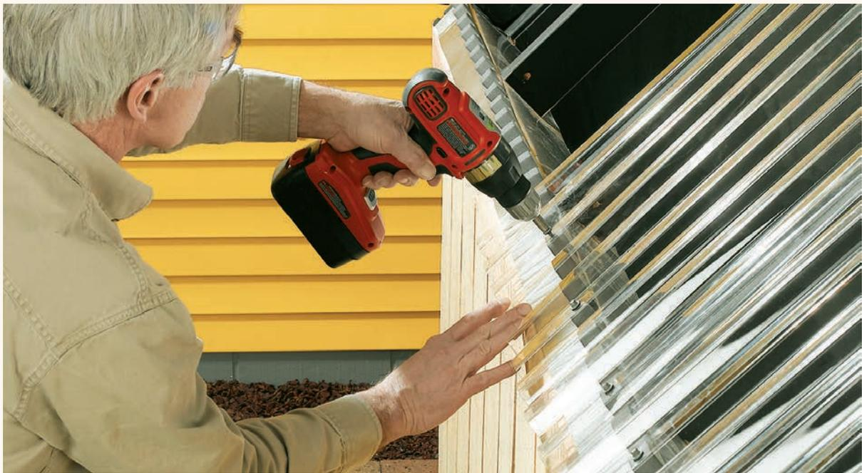
**21** Set the panels in position over the foam closure strips, then predrill the holes on the crowns. Use a sharp bit  $\frac{1}{8}$ " bigger than the diameter of the neoprene screw to allow for movement. Don't overtighten the screws—they should be tight against the panel, but should not distort it.
