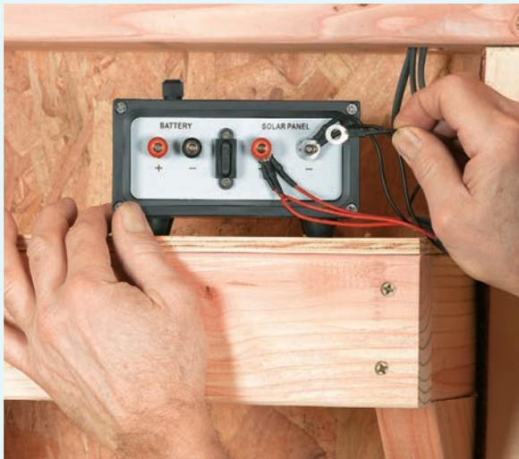
**8** Connect the wires from the PV panels to the solar terminals on the back of the regulator/charge controller. Secure the wires to the walls or roof framing members to keep them clear. *CAUTION: The collector panels should be covered with a drop cloth or opaque material well before making these connections. Tape or clamp the drop cloth so it doesn't blow off.*
