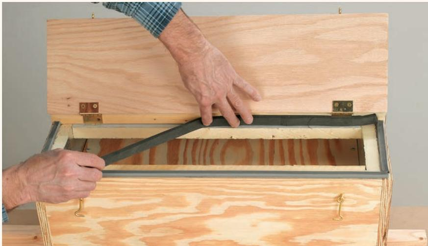
**14** Cut 1 × 8s to fit for covers for the inlet and outlet, so that heat won't be lost when the sun goes down. Apply self-adhesive weatherseal around the edges, then screw on two or three hinges, depending on the width of the window. Use hooks to hold the upper cover in place and small barrel bolts to hold the lower cover.
