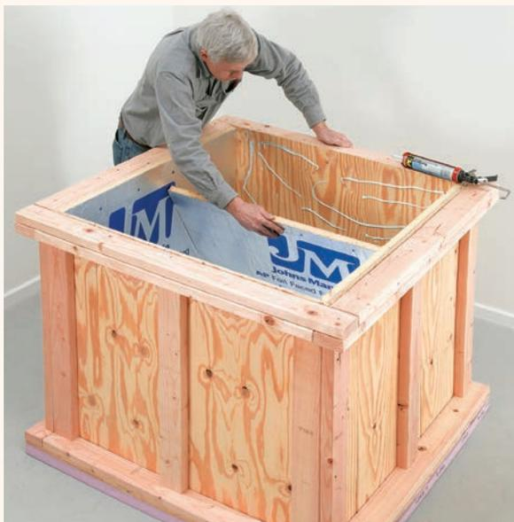
**7** Place the polyiso insulation inside the box, using the foamboard adhesive to attach it. You don't need much; the water will hold the insulation in place. Add the second layer, then seal all the corners on the bottom and sides with silicone caulk.
