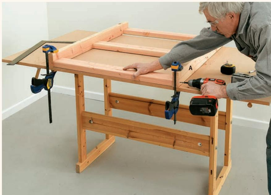
**1** Screw two of the 41" 2 × 4s to three vertical 2 × 4s, then fasten the 41"-wide piece of ½" plywood to the 2 × 4s with construction adhesive and 1½" screws. Repeat for the opposite side. Align the bottom edge of the plywood with the bottom 2 × 4; the top edge will overhang 1½".
