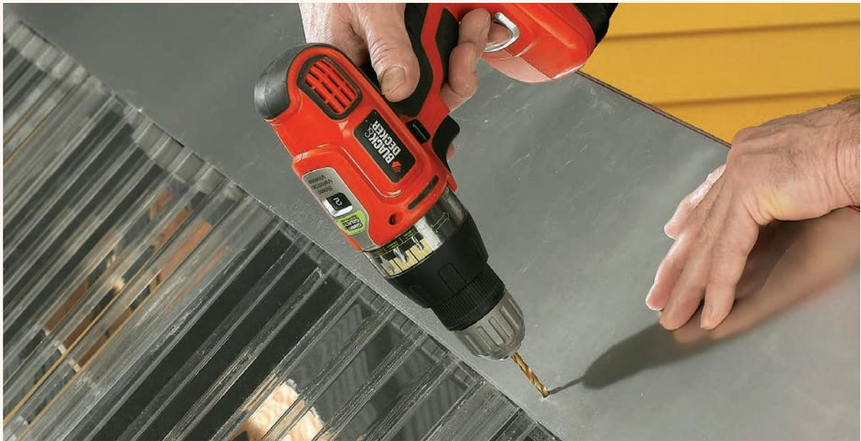
**22** Cut a 14"-wide piece of sheet-metal or aluminum coil stock slightly longer than the roof, then bend it at the center to create a cap for the roof. Drill holes through the metal, polycarbonate, and closure strips in the front, then fasten with neoprene screws into the blocking. Screw the metal to the 1 × 6 in back.
