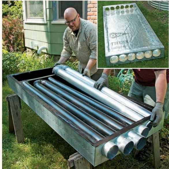
**10** Insert the ductwork. Beginning at the inlet duct, guide 4" aluminum HVAC ductwork in a serpentine shape throughout the entire multi-panel installation, ending at the outlet duct. Join ends of adjoining duct sections with flexible duct connectors fashioned into a U shape and secured with metal screws and foil tape. Paint each section of ductwork with black high-temperature paint once it is in place.
