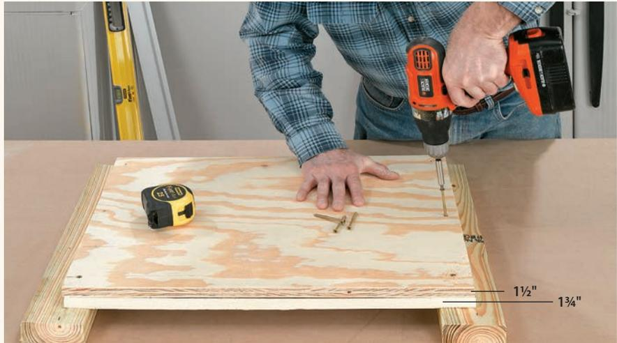
**3** Screw the first layer of front and side pieces to the base and to each other, then add the back piece. Pre-drill the screws with a countersink bit.
