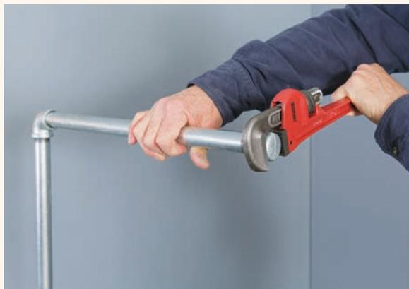
**14** Assemble the cooking stand with prethreaded steel pipe and fittings. Thread two 18" pipes into the two side outlets of a 3-way fitting to form the stand base. Tighten the connections with a pipe wrench. Add caps to the ends of the pipes. Thread a 42" pipe into the top outlet of the 3-way, extending up. Add a 90° elbow to the top vertical pipe and then a 20" pipe outward from the elbow. Slip an S-hook onto the 20" pipe, then add a cap.
