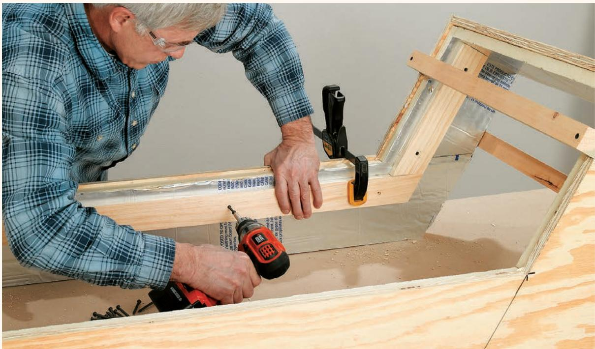
**5** Screw the 1 × 3 nailers to the sides of both the long and short pieces using 2¼" screws. Place the nailers 1¼" from the bottom edge to leave room for 1" insulation and ¼" plywood.
