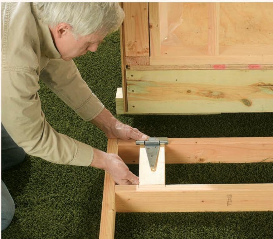
**11** Frame the rear doors. Make sure that the doors are  $\frac{1}{2}$ " less than the height of the opening and  $\frac{1}{2}$ " less (total) than the opening width. Frame openings for the vents, and add a hinge backer.
