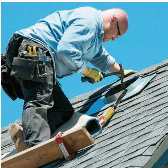
**15** Use a roof jack to form an 8"-dia. opening. Apply a heavy double bead of roofing cement along the top and sides of the jack. Nail the perimeter of the flange using rubber gasket nails. Cut and install shingles with roofing cement to fit over the flashing so they lie flat against the flange.
