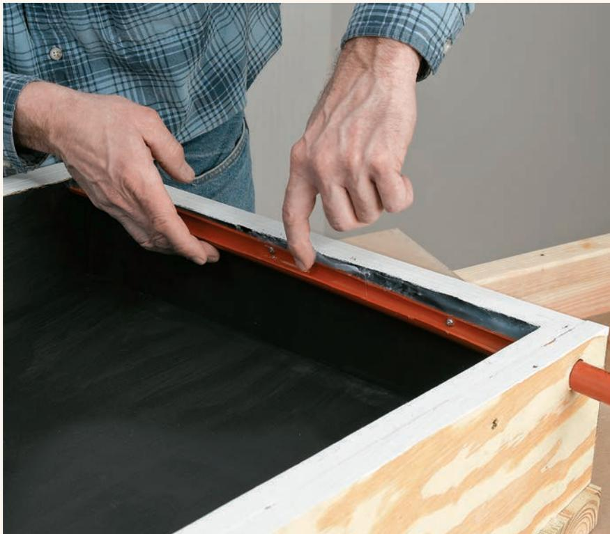
**11** Wipe a thick bead of silicone caulk along the top edge of the PEX to seal it against the plywood.
