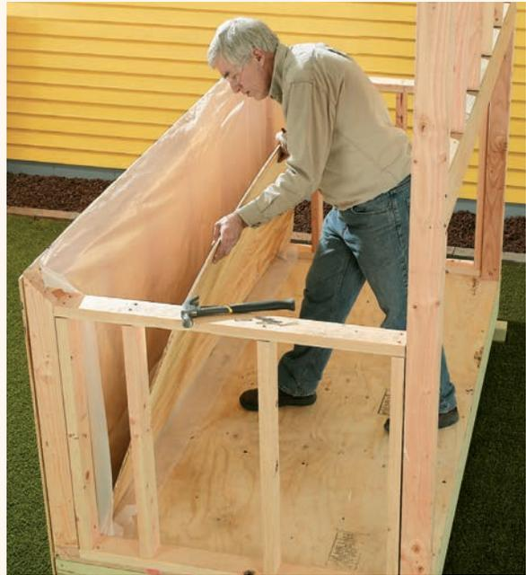
**7** Insulate the front wall, then add the vapor barrier and the  $\frac{3}{8}$ " interior plywood siding. Leave the plywood  $\frac{3}{8}$  to  $\frac{1}{2}$ " short of the top plate.
