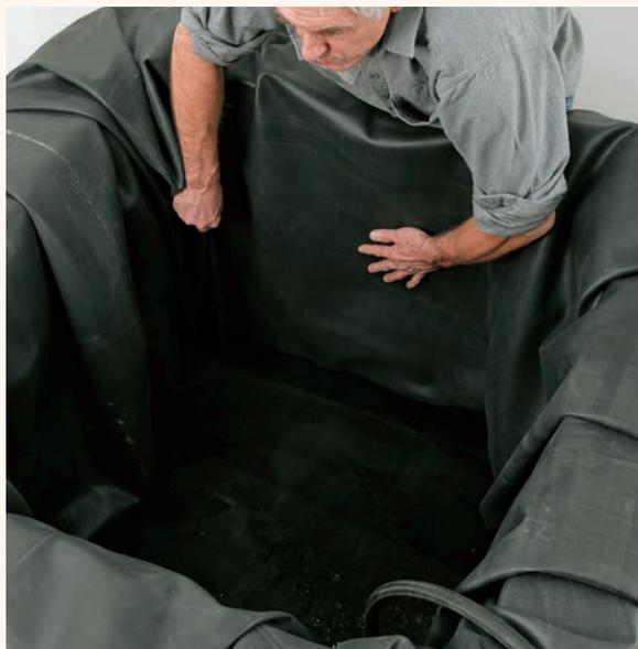
**8** Cut and set aside a 5 × 12' piece of the EPDM for the top, then fold the remainder into the tank. Work it into the corners, leaving the rubber loose at the bottom so it doesn't stretch with the weight of the water. Add 6" of water to hold the rubber in place as you fold over the corners. Drape the excess over the sides.
