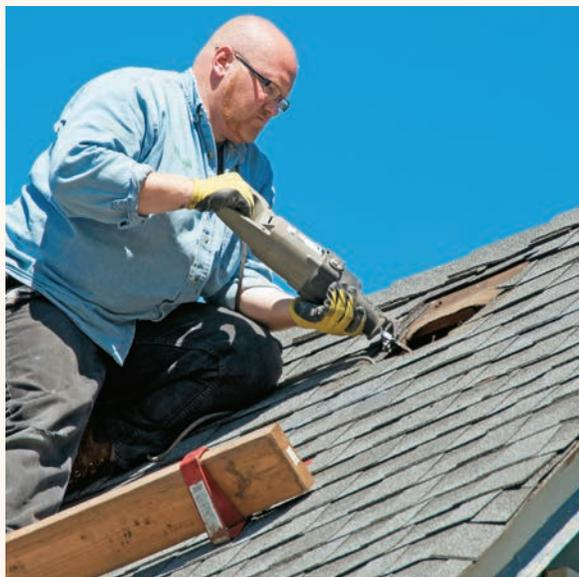
**14** Mark off the panel layout locations on the roof. Transfer the locations of the 8"-dia. inlet and outlet holes to the roof as well. The location of these holes should not interfere with the structural framing members of your roof (either rafters or trusses). Adjust the panel layout slightly to accommodate the best locations of the inlet and outlet, according to your roof's setup. Cut out the inlet and outlet holes with a reciprocating saw.
