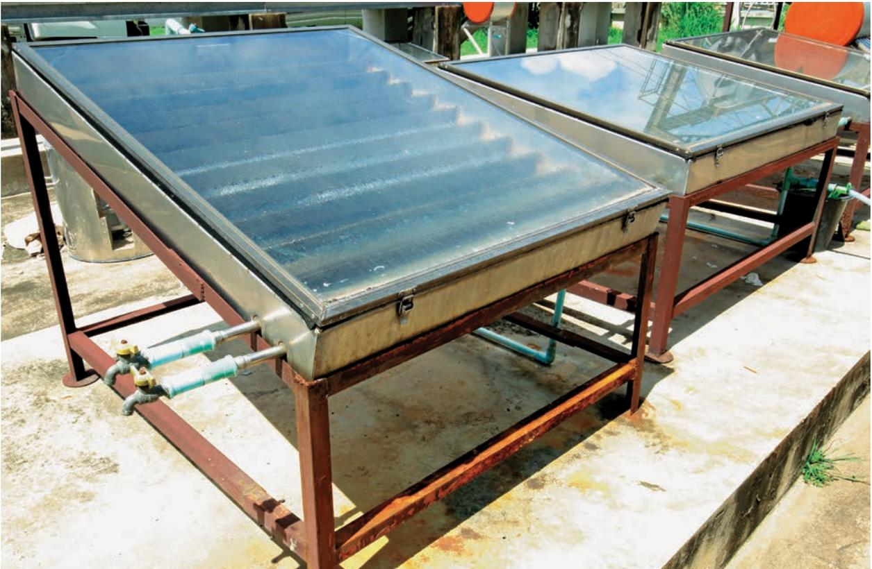
Solar water heating systems can heat water for domestic use (drinking, showering, etc.) or for water-based space heating systems. In both cases, the solar system typically preheats the water and a conventional water heater or boiler takes it from there. Commercial hot-water systems (top) save fuel, although the cost savings vary. DIY systems (bottom) can offer better payback potential.
