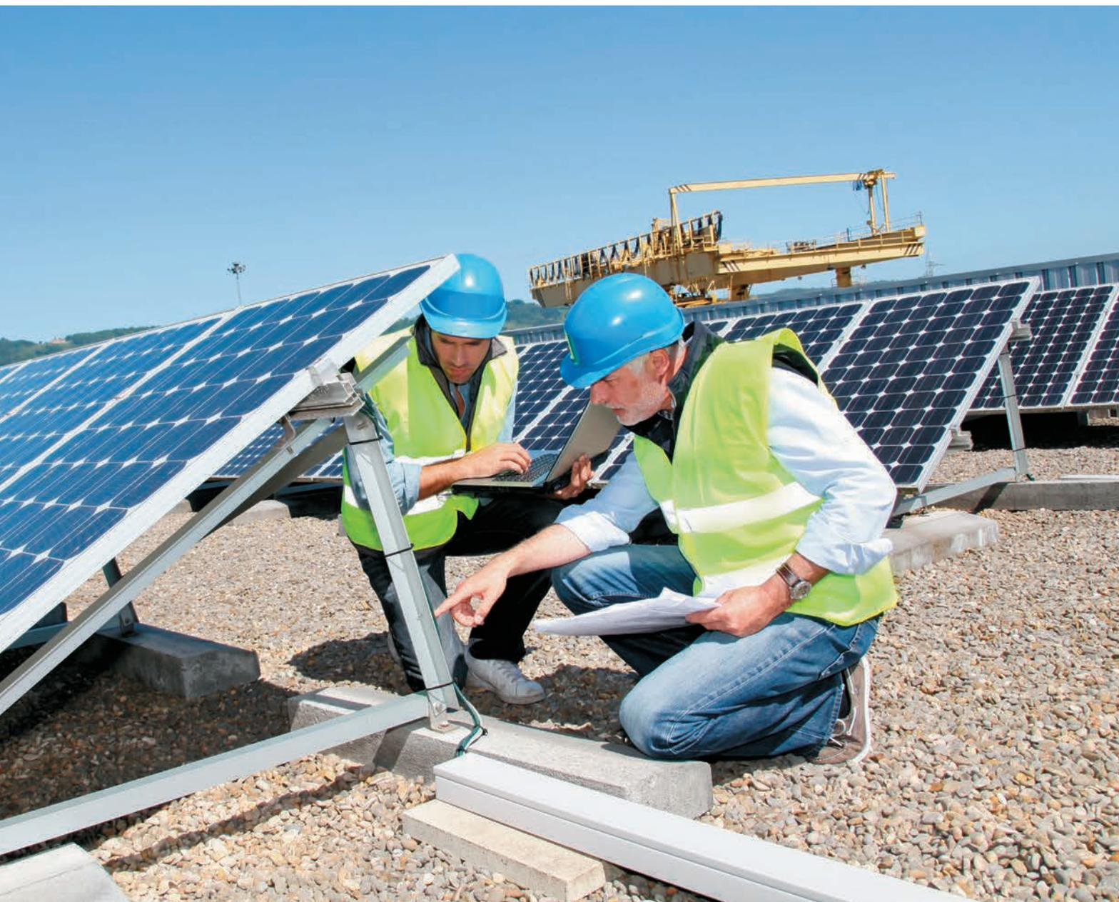
Rooftop mounting systems are made with lightweight, corrosion-resistant metal (typically aluminum), and should last at least as long as the modules. Many mounting systems are designed to work with different brands and sizes of modules.
