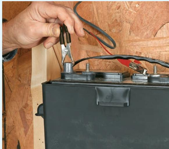
**9** With the regulator turned off, fasten the battery leads to the back of the regulator, then clamp them to the battery posts—black to negative first, then red to positive. Then uncover the PV panels. Double-check the connections, then turn the regulator/charge controller on. For a 12V battery, the voltage output reader will show 13 when the battery is fully charged.
