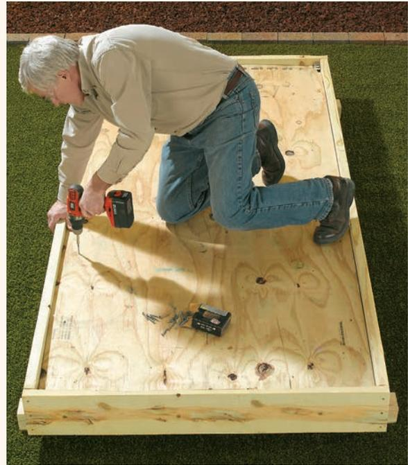
**2** Flip the framework over, then screw 1/2" treated plywood to the underside of the frame. Caulk all the edges to prevent ants and other insects from colonizing the base.
