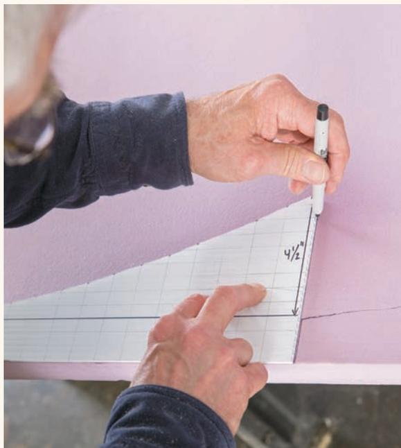
**6** Trace around the template to draw 16 ribs onto  $1\frac{1}{2}$ " rigid insulation board, using a fine marker. Cut out the ribs with a jigsaw.
