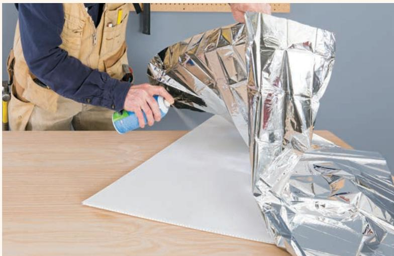
**5** Cut the Mylar sheeting by placing each reflector panel facedown onto the backside of the Mylar and cutting the Mylar around the panel, leaving an ample margin on all sides. Turn the panels face up and coat them with spray adhesive. Apply the Mylar to the panels so it is smooth and flat, then bend the excess over the backside of the panels and glue in place with spray adhesive.
