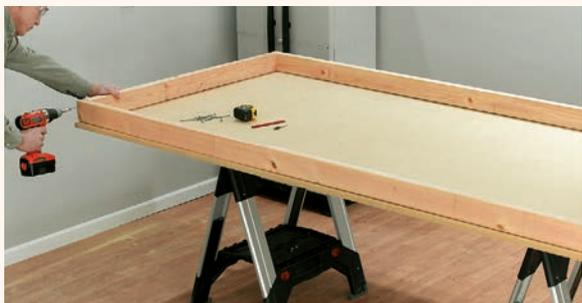
**1** The frame that houses this solar water heater is constructed from 2" × 4" and 2" × 6" dimensional lumber. Cut the pieces of the frame to length, then join them with 2½" deck screws driven into pilot holes.
