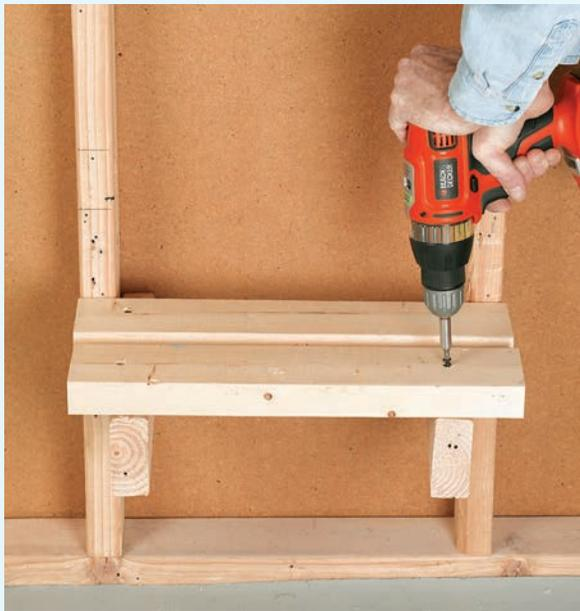
**9** Build a support shelf for the battery using 2 × 4s. The shelf should be at least 18" above ground. Set the battery on the shelf in a sturdy plastic case.
