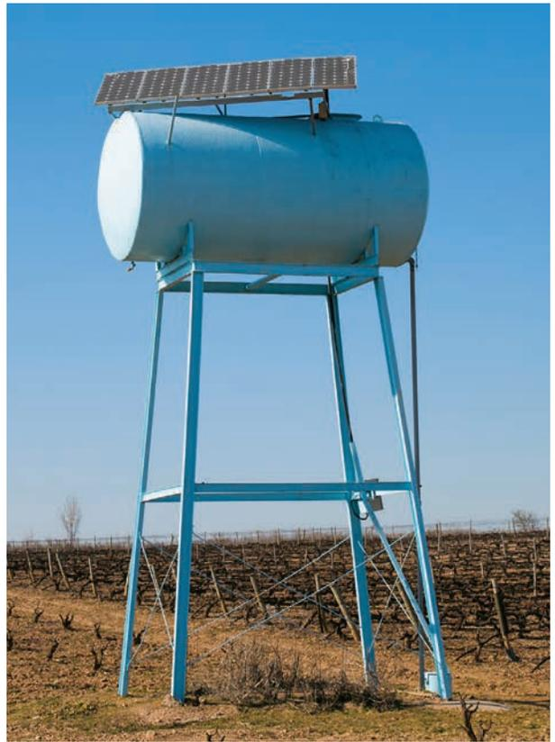
Water for irrigation is continuously pumped from a deep aquifer up to this storage tank during the day as long as the sun is shining.
