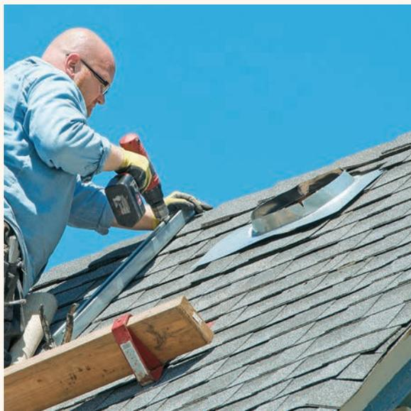
**16** Attach Unistrut mounting U-channel bars to the roof for each panel. Use the chalklines on the roof to determine the position of the Unistrut, and attach to the roof trusses with Unistrut connectors.
