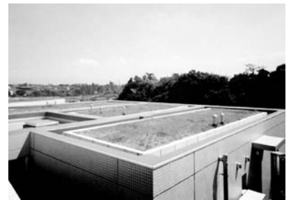
6.17 Earth roof system of the eco-village, Matsudo, Japan
