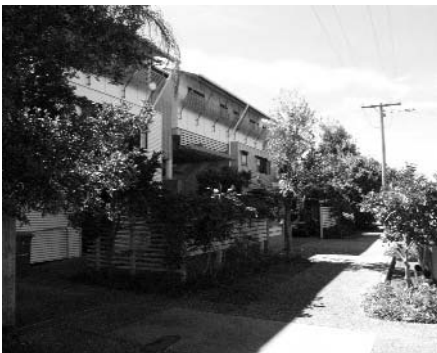
7.21 Cotton Tree Housing: south (polar-facing) façade. Three storey units are placed to the southerly zone on the site to facilitate ventilation to the northern zones
