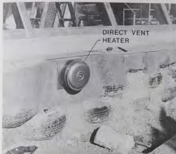
A direct vent heater through the front face tire wall shown above.
