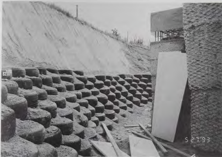
TIRE RETAINING WALL BEHIND EARTHSHIP IN JAPAN.
