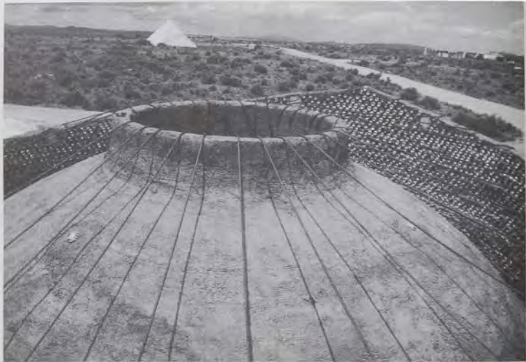
FORMING THE INSULATION CAVITY OF THE CAN DOME
