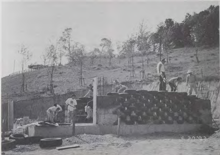
EARTHSHIP IN JAPAN UNDER CONSTRUCTION SHOWING KNITTED IN CONCRETE COLUMNS
